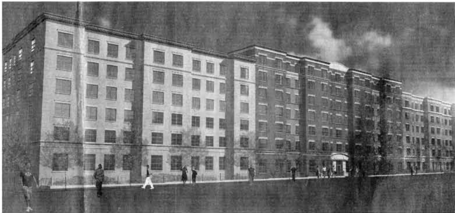
ABOVE: This 150-unit mixed-income development is planned for a vacant lot at 1825 Atlantic Ave. at Suydam Place in Bedford-Stuyvesant. LEFT: This 10-story, 80-unit co-op building, to be called Atlantic Terrace, is planned at 669 Atlantic Ave., between South Portland Avenue and South Oxford Street in Fort Greene.
